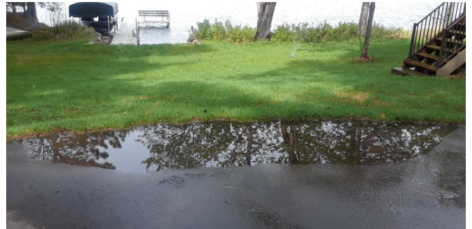
Berm Along Driveway Edge
